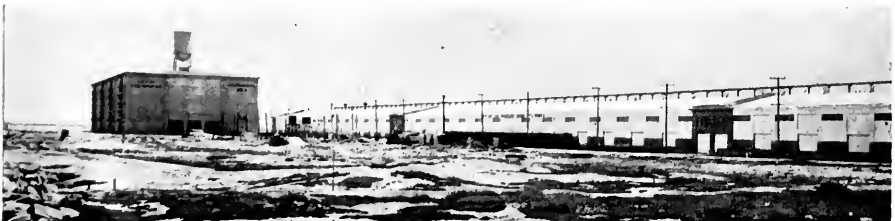
Steel freight shed, 1800 feet long, 100 feet wide, on the westerly side of municipal pier No. 1. This is an earth-filled pier, 650 feet wide and one-half mile long. The transit shed is on a reinforced concrete wharf with 600 feet of open wharf at the northerly end not shown in the picture. At the extreme left is municipal warehouse No. 1, showing its relation to the transit shed.
